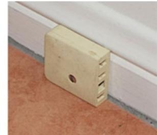
This is one of the most common technology on old residential or commercial areas. The optic fibre is delivered to a distribution point in the street and then is delivered with copper to the first socket of the premises.
